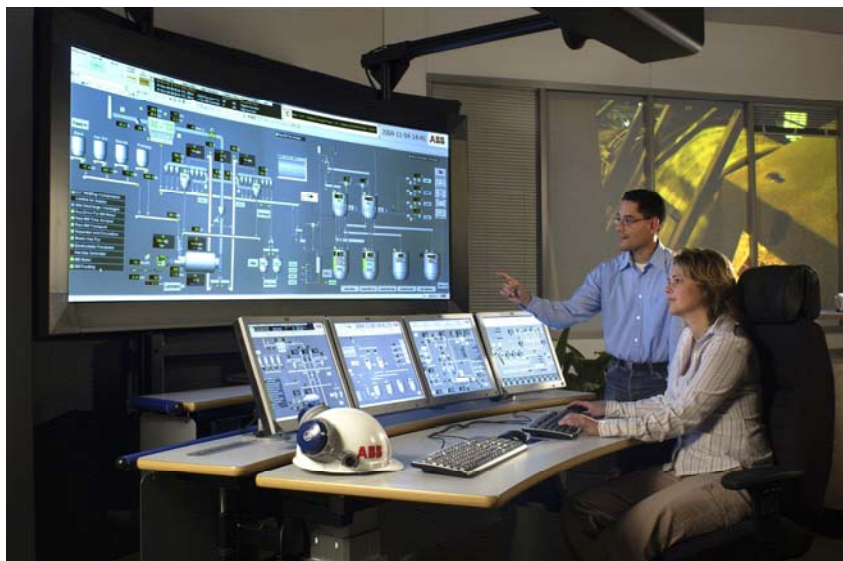
Fig. 5: Enhanced display facilities that can be further developed (courtesy ABB)
